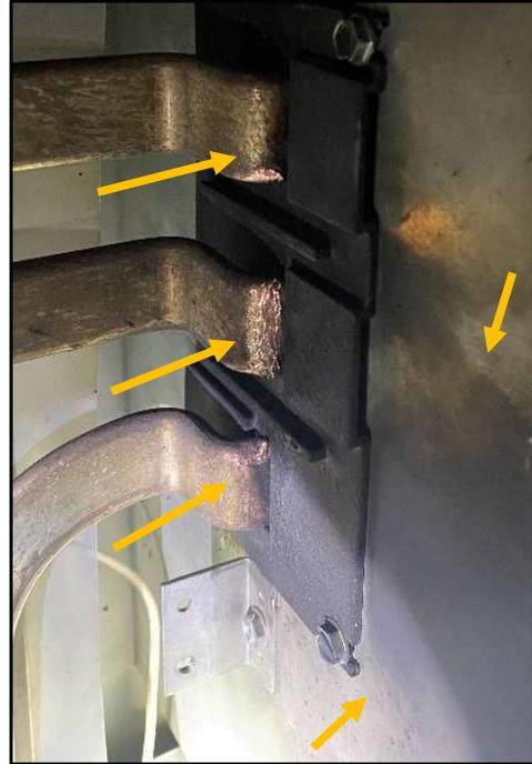
Fig. 12. Damaged bus bars in 1200A CB cabinet.
